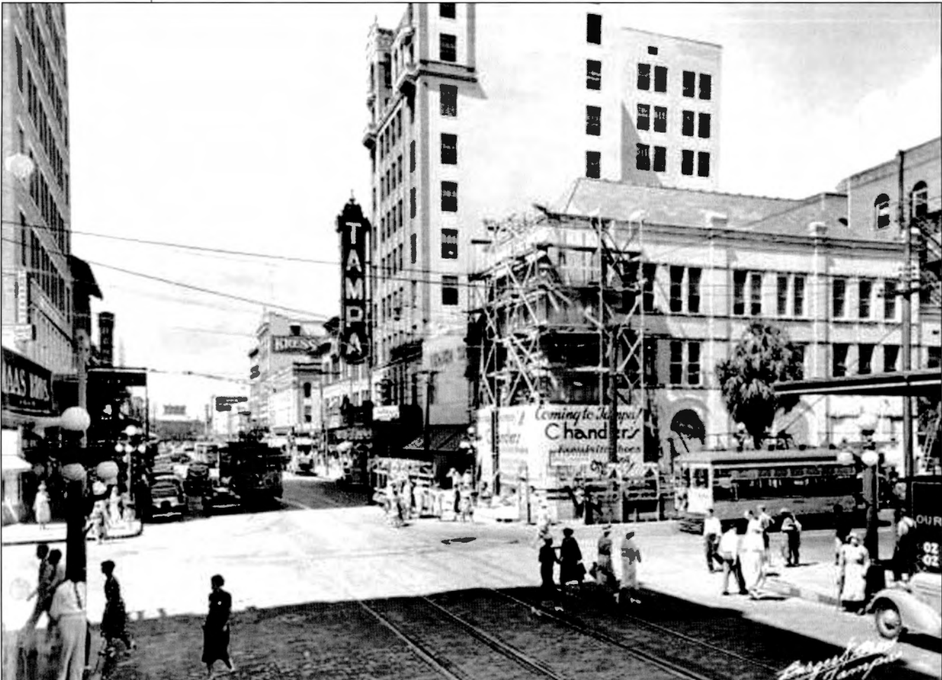
A view of a very busy Franklin Street looking north from Zack Street. Two streetcars are approaching the intersection and the Tampa Theatre is on the right in the next block. Construction on the facade of the First National Bank can be seen. (Courtesy of the Burgert Bros. Collection, Tampa-Hillsborough County Public Library.)
